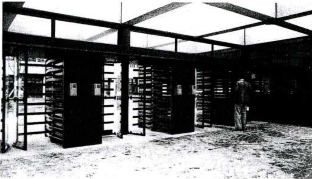
Fig. 15 Supervised entry zone of an administrative building of the Swiss Confederation. The revolving doors will only be opened, when the access control readers ID 2000 have identified the authorization of access.
